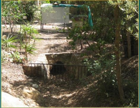
(Properly) install & maintain debris racks upstream of drains
