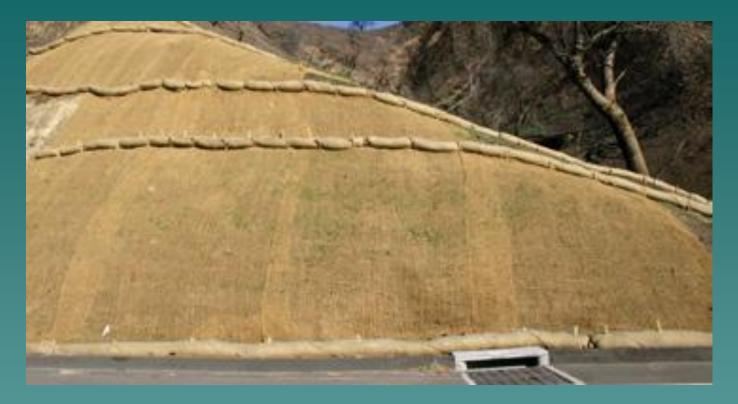
The best protection for this slope is to get grass growing on it. The jute blanket protects seed & seedlings from rain-drop impact & sheet erosion. Straw-rolls or Waddles slow down small flows of water & detain small amounts of sediment.
